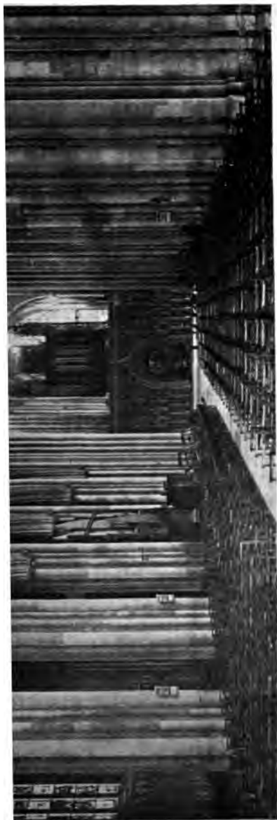
NAVE, LOOKING EAST Cathedral, York
